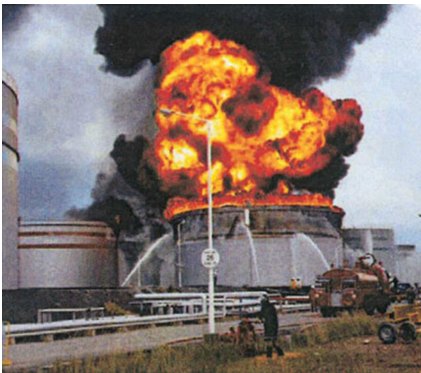
Fig. 5. Ignition of the second tank due to radiant heat [23].
