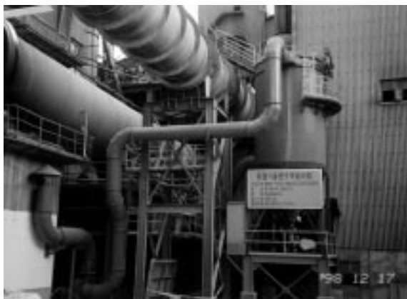
Fig. 3. Photograph of CYBAGFILTER of 18,000 m 3 /hr capacity. (a) Magnification 773X (b) Size distribution.
