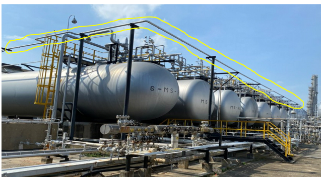
Fig. 4. Water curtain of ammonia tank.
