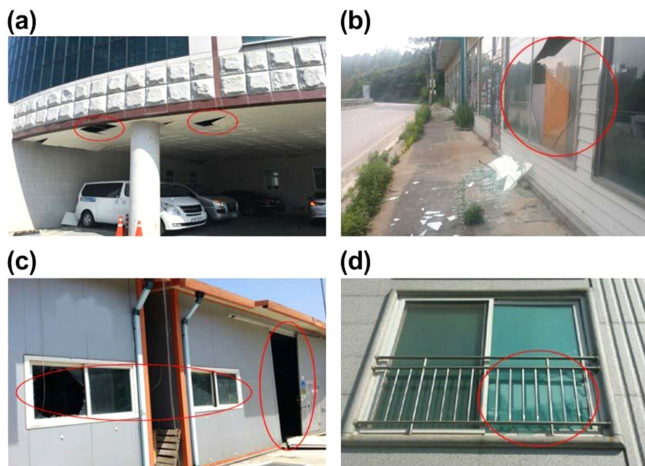
Fig. 4. (a) Damage to Building No. 1, disassembled ceiling; (b) Damage to Building No. 2, broken door and window; (c) Damage to Building No. 3, distortion of frame (beam); (d) Damage to Building No. 4, broken door and window.
